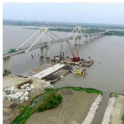
Pumarejo bridge - Barranquilla - Colombia
