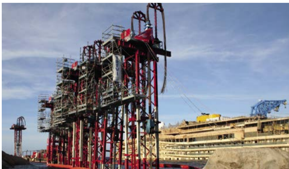
Costa Concordia recovering project. (ph. credit Trevi)
