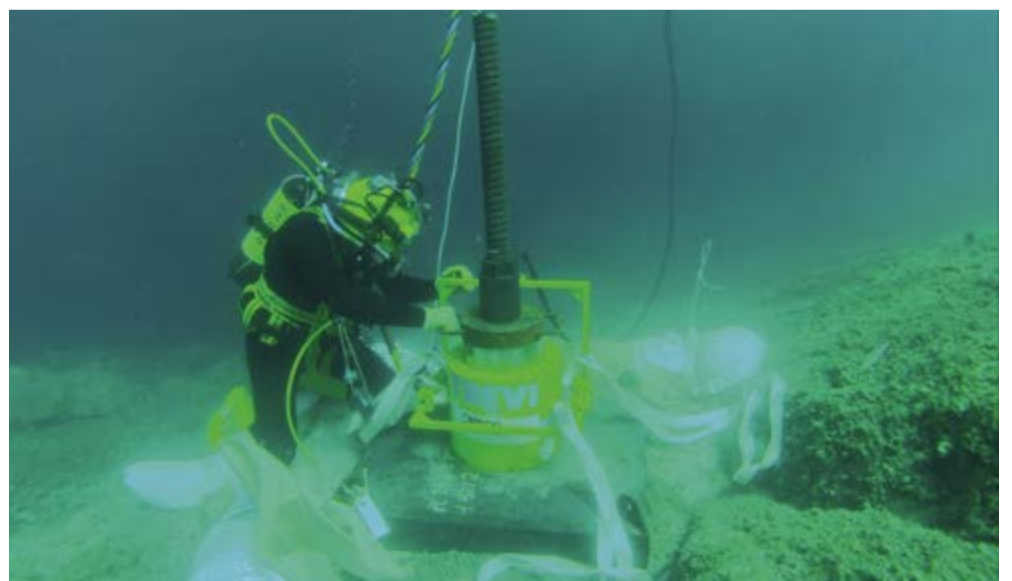
Underwater preliminary anchor tension tests, up to 290 Ton. (ph. credit Trevi)
