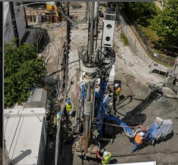
coring to be executed on 5% of the installed columns. At intervals of 3.0 ft. of vertical treatment, soil-cement mixture was tested for unconfined compressive strength (UCS) and hydraulic conductivity (HC) and the 28-days results needed to comply with the minimum design criteria of 100 PSI and  $1 \times 10^{-6}$  cm/s respectively.
