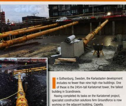
clay soil, meaning the sheet-piled retaining walls require support ahead of the basement slab being cast. Due to the irregular heights of the basement sides, Groundforce braced the retaining walls
