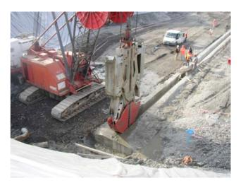
The trench, maintained full of biodegradable mud, was excavated continuously. The biodegradable mud, made of water and natural polymers (poly-saccharide), was batched at site using an apposite mixing plant.
