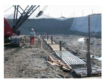
At the completion of the casting works, the degradation of the polymeric mud remaining in the trench was accelerated, by circulating specific enzymes through pipes installed in the trench on purpose.
