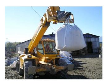
The trench was backfilled with reactive material up to the max elevation reached by the groundwater table excursion (2 m from working platform). The zerovalent iron was imported from Germany in big bags (2 ton). It is constituted by 0.2-3.0 mm particles, absolutely free from oils or other impurities. At all times during the work activities, great care was paid to avoid/reduce its contact with air, in order to prevent the iron oxidation.
