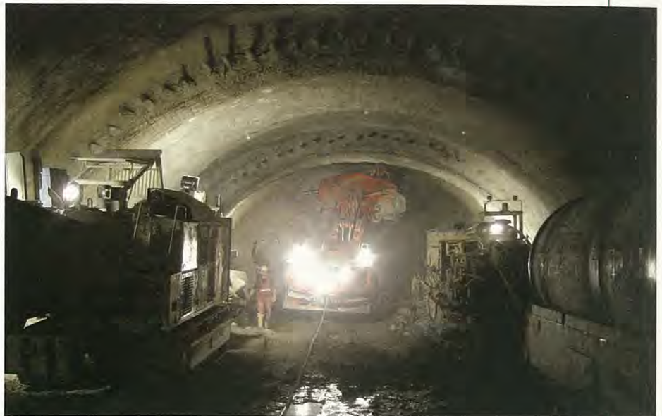
Above: Grouted tube stabilisation was used substantially in loose ground
