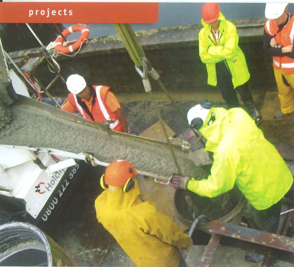
LEFT: Pouring slot for concrete using a tremie pipe. ABOVE: A line of pre-drilled holes five metres deep.
