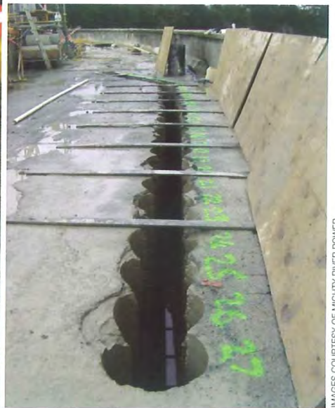
LEFT: Pouring slot for concrete using a tremie pipe. ABOVE: A line of pre-drilled holes five metres deep.
