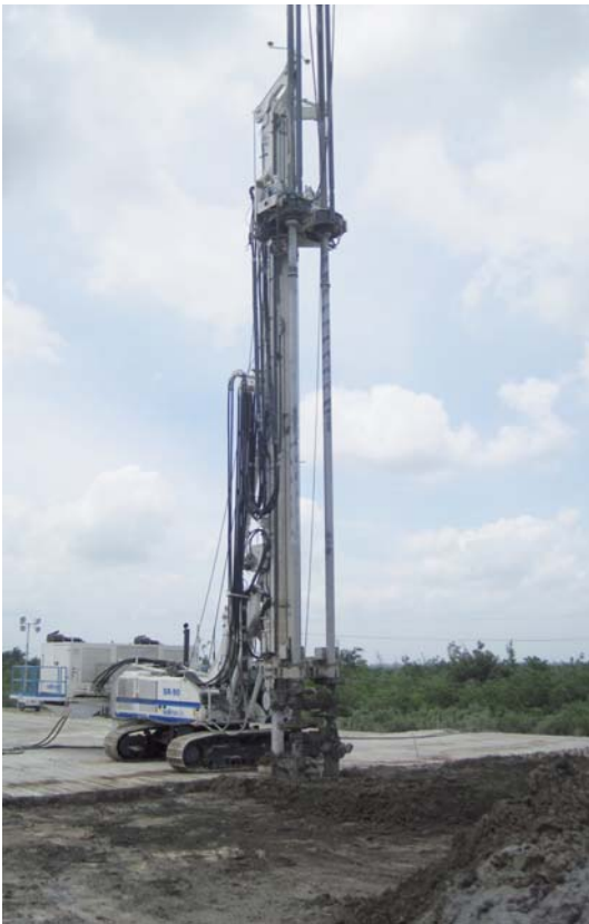
STEP 1 Drilling and simultaneous treatment with high-pressure injection of cement grout
