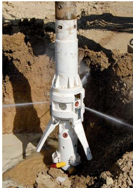
Turbojet tool to install bottom slabs
