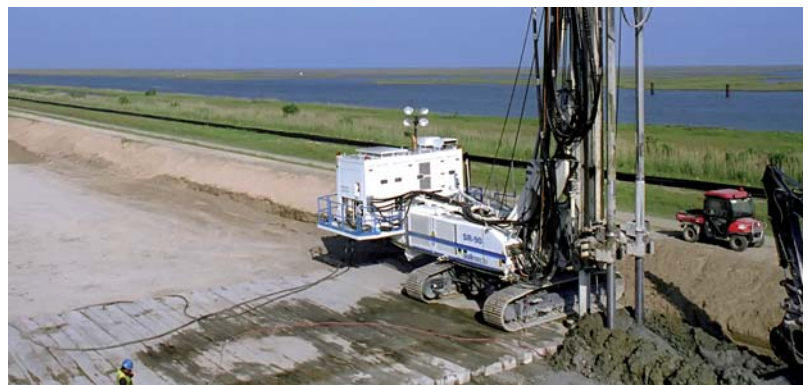
STEP 2 Uplifting and simultaneous treatment with high-pressure injection of cement grout
